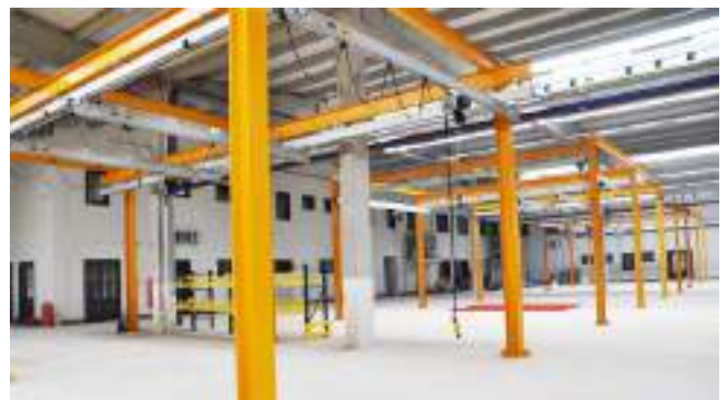
Workstation cranes with chain hoist
